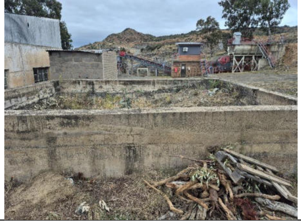
Cleaned storage area
