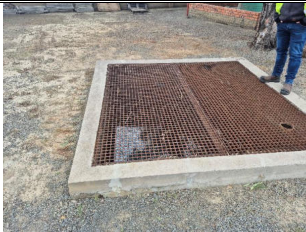
Bund of hazardous waste area to be sealed
