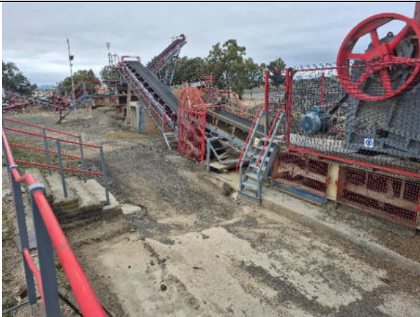
Plant area neatly managed
