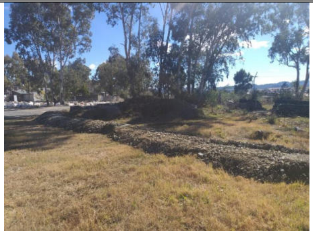
Stormwater berms in place
