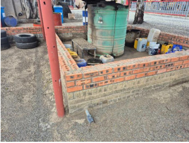
Bund of hazardous waste area to be sealed
